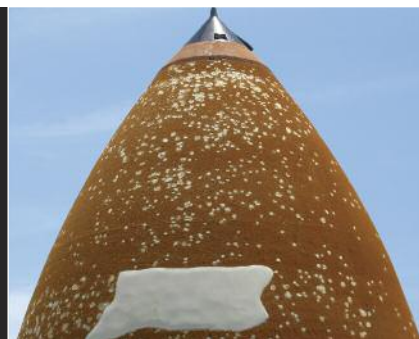
ET-124 damage repairs, post storm.
